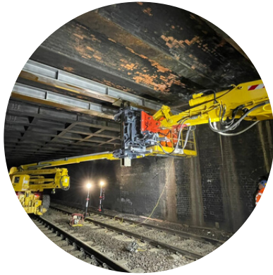
Replacing the life expired steel supports in the tunnel
